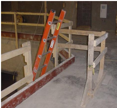
Use offset to protect ladder opening
