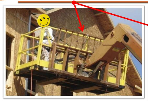
Fall Arrest Anchorages shall be capable of supporting at least 5,000 pounds per employee
